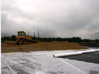
intermediate layers of fill would be necessary to deliver the required load-bearing capacities for each of the elements. In addition, the individual layers were separated by nonwoven geotextiles, also provided by Bonar.
