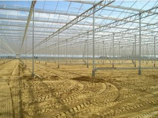
Nowadays, 5-axle, 60-ton trucks may drive, unidisturbed, in an area of former marshlands, where a major greenhouse complex was built on a floating foundation. New economic value - thanks to the outstanding stabilizing properties of Enkagrid.
