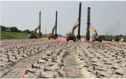
Little flags mark the installation location.
