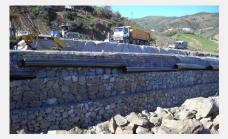
Enkagrid layers pending the levelling and compaction of soil layer
