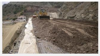
Levelling/compaction of the filling, gabions being used as well as temporary formwork, Enka-Tex pending layer on the gabions
