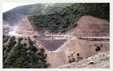
Enkagrid retaining solution minimised the load on top of the existing slopes
