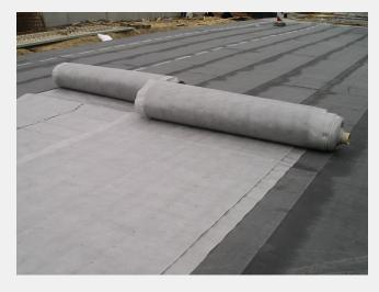
The large size of the Enkadrain rolls enabled a speedy installation of the drainage system on the deck.
