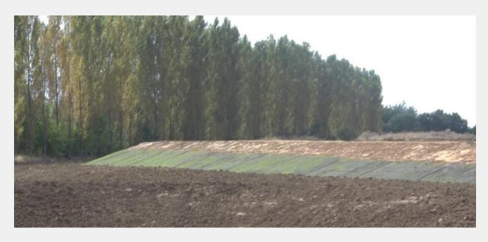
The embankment was built with locally available soil with sufficient germination potential. However, because of the possible breakthrough of the reservoir dam, a huge water flow can be expected that is guided along the new dyke, causing considerable damage.
