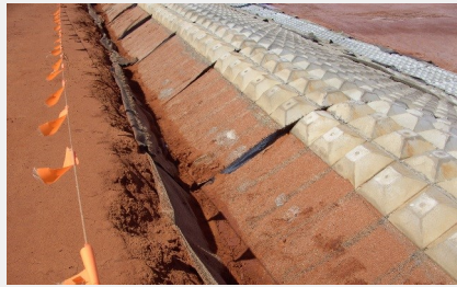
The anchorage trench was filled with concrete
