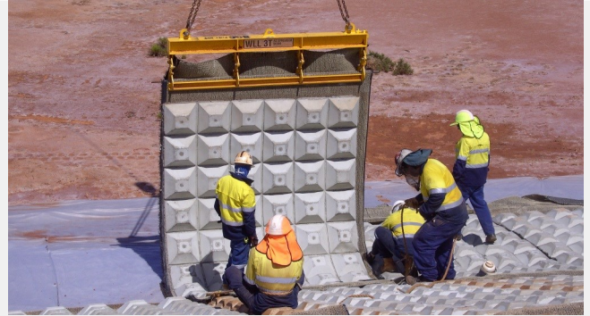
Installation of the product
