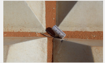
The panels itself were fixed with metal pins
