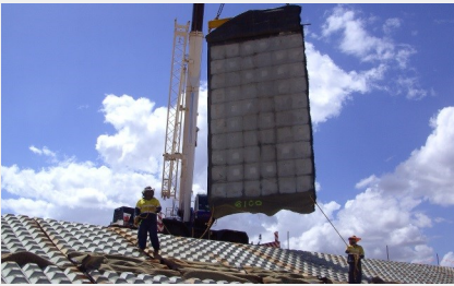
Enka-Fix is strong enough to lift the concrete mats in the air
