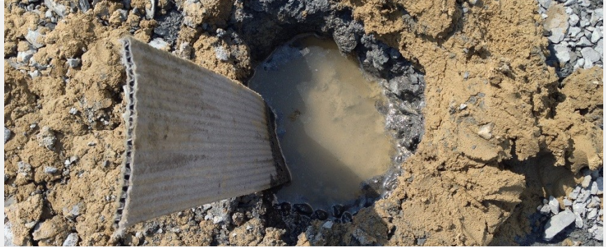
Colbondrain CX1000 - at work
