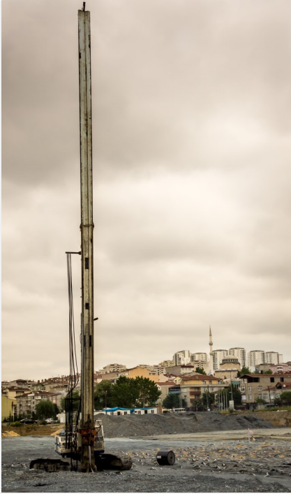
Installation machine installing Colbondrain CX1000
