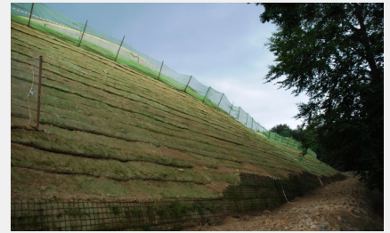
Finished outward slope of embankment (inclination 47°) with installed erosion control
