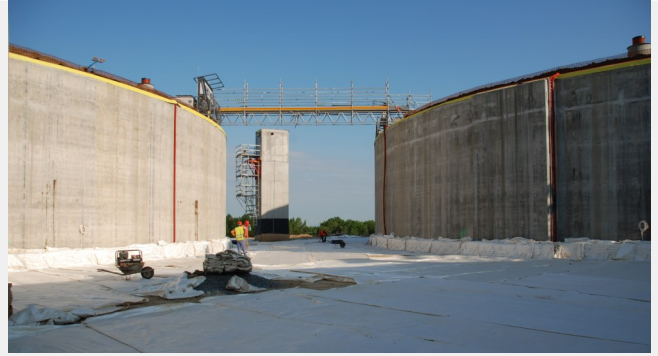
Installation of the geosynthetics between the tanks
