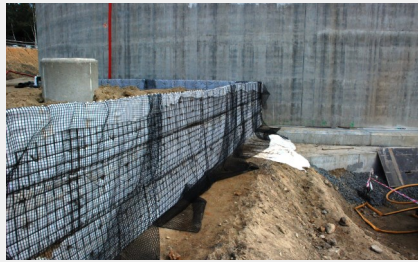
Detail of the wrap-around facing supported by a steel mesh formwork
