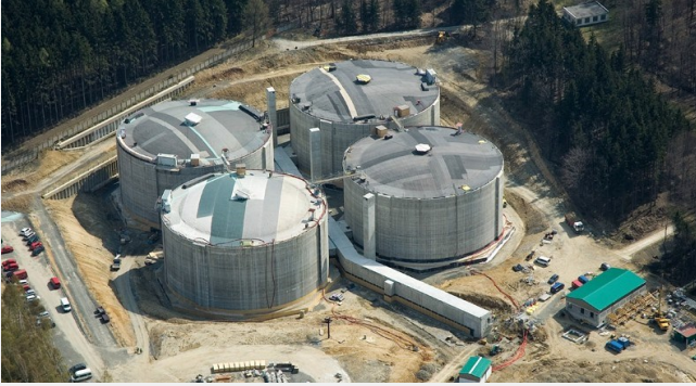
Construction works and technology in place before the earth works phase
