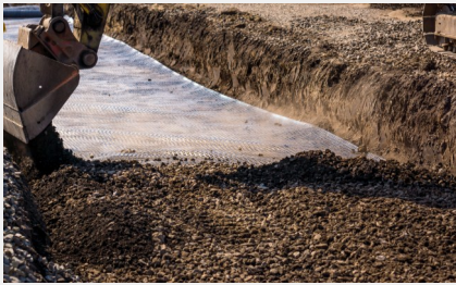
Filling the granular sub base material
