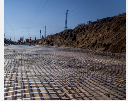
Installation of the Enkagrid MAX 40
