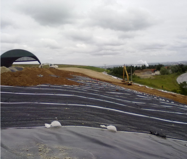
General view of the refurbishing area
