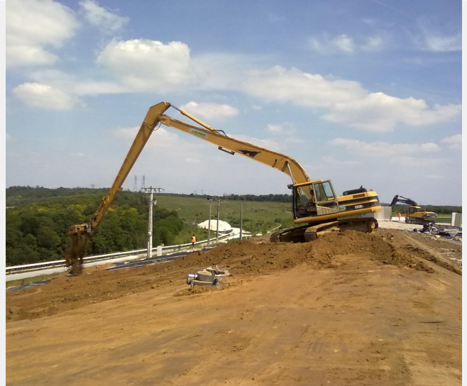
Covering soil installation with long shovel Caterpillar 325 BL
