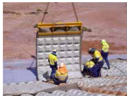
Installation of the product
