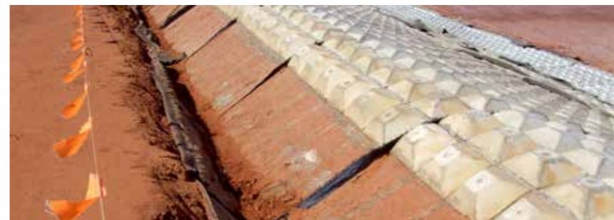
The anchorage trench was filled with concrete
