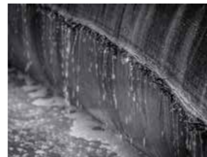
Water coming out of the Enka-D-Tube is very clear.
