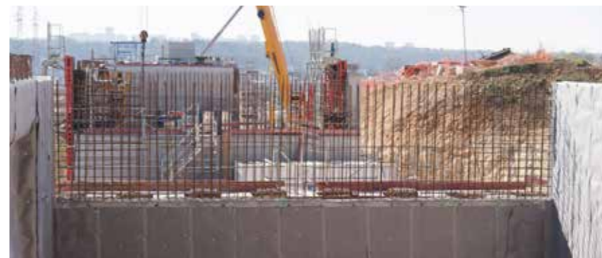
No loss due to overlapping: Enkadrain is provided with 10 cm overlap of fleeces
