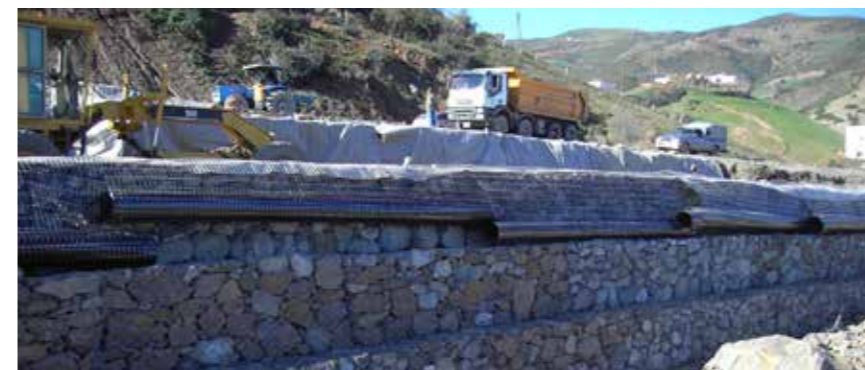
Enkagrid layers pending the levelling and compaction of soil layer
