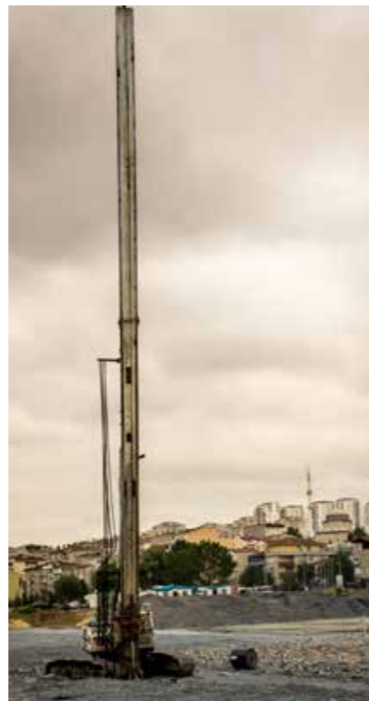
Typical installation rig for Colbondrain CX1000
