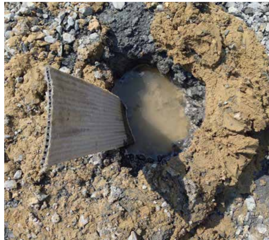
Colbondrain CX1000 - at work
