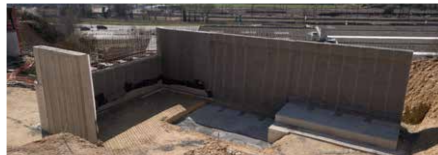
Overview of the abutment
