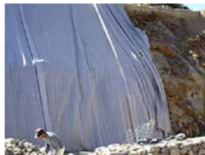
Harsh conditions require an Enkadrain with high tensile strength and puncture resistance
