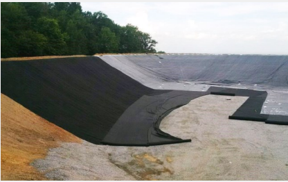
Installation works: Enkadrain is laid underneath EPDM geomembrane
